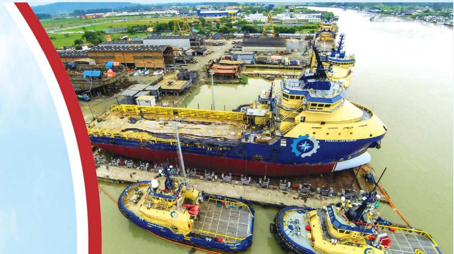
Dry dock – 110m Length, 23m Breadth and upgraded capacity for 5200 T
