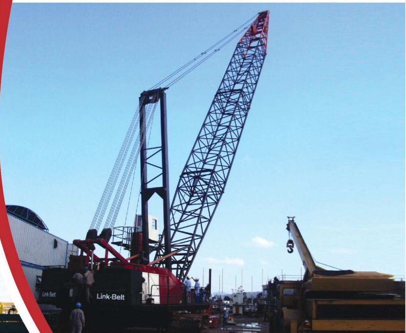
3 crawler cranes 02x 250 T and 01x 450 T
